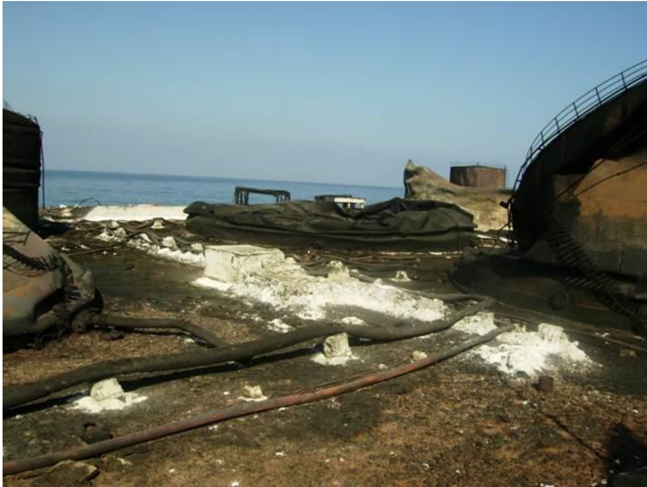
Closer view of a collapsed tank within the storage facility
