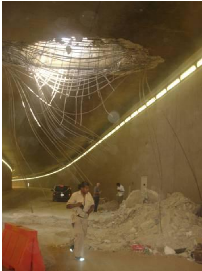
Wider view of damage to underside of runway
