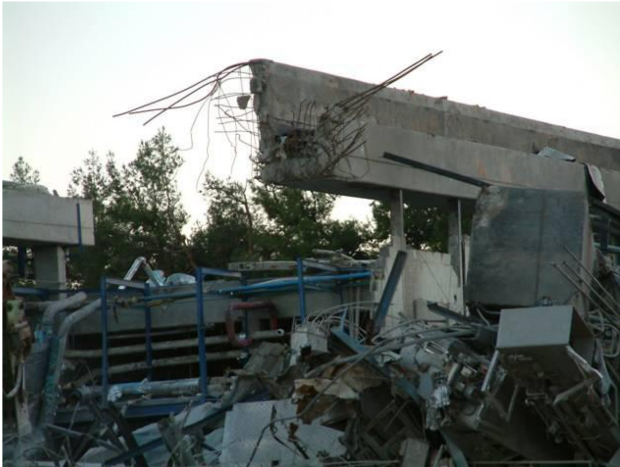
Damage to reinforced concrete supporting beam
