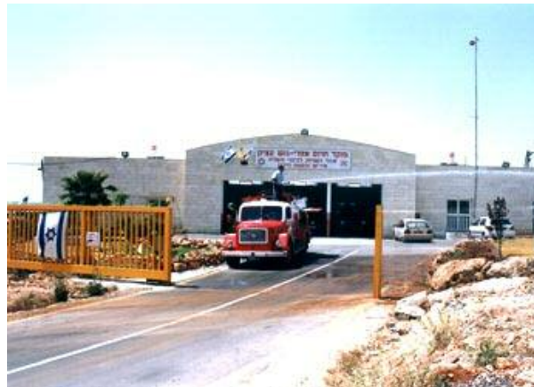
Regional Rescue, Fire and Trauma Station (La Mizrak)
